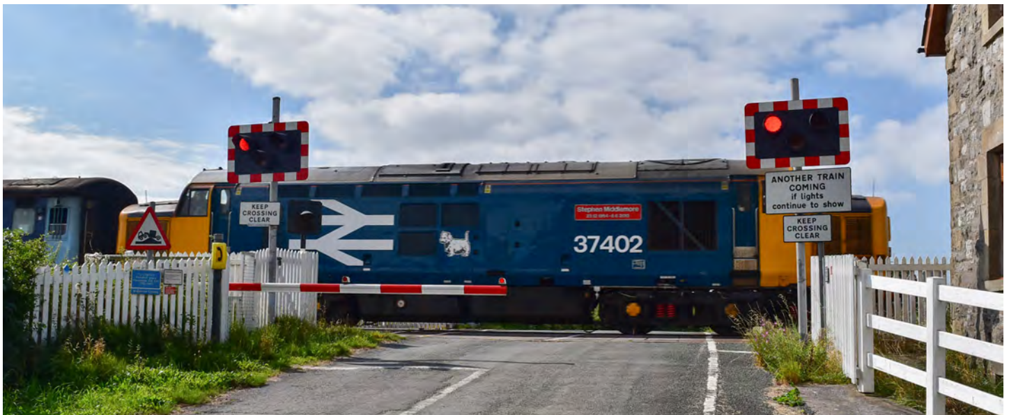
Figure 6 – AOCL+B crossing installation at Wraysholme level crossing in Cumbria, UK.
