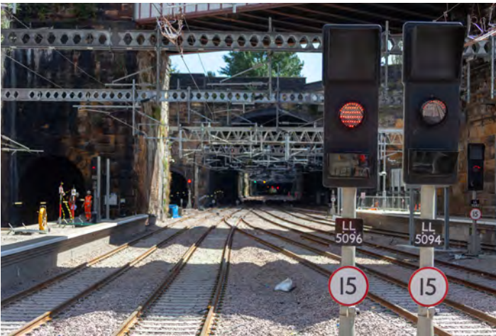
Top, new signals and their supporting gantries before being brought into use at Liverpool Lime Street. Above left, a view along the station throat. Above right, testing at Manchester Rail Operating Centre. All photos Matthew Nichol Photography.
