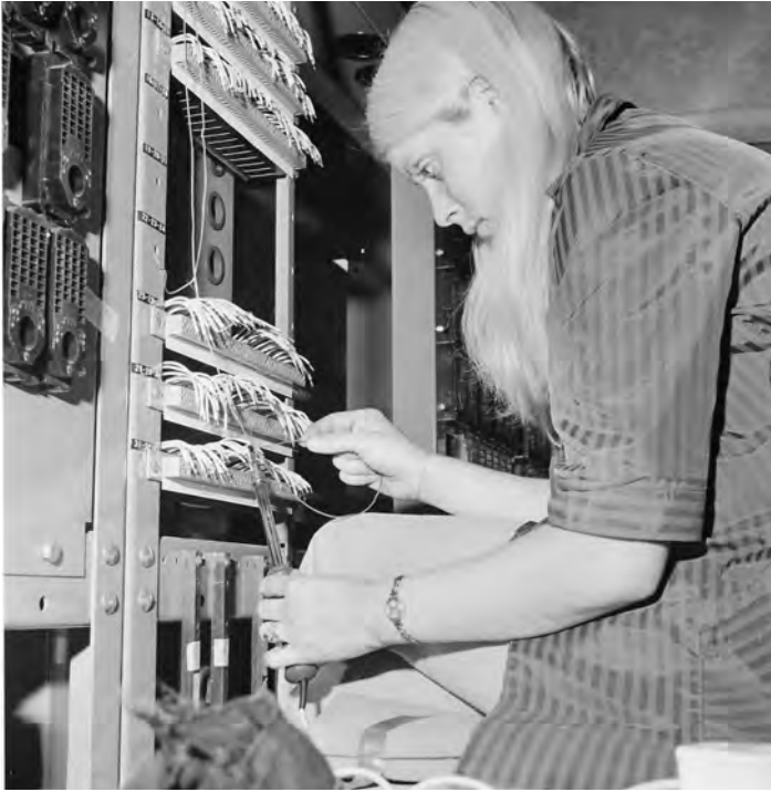
Terminating connections at Warrington PSB, 1972.
