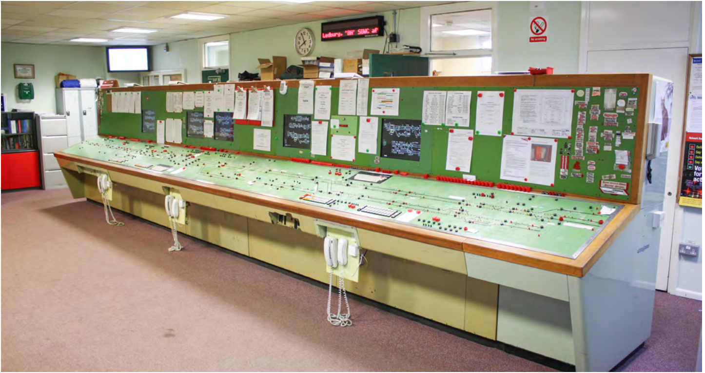
The control panel at Swindon, originally commissioned in 1968 and based very much on the standard 'turn and push' control panel design adopted as part of the WR RRI project. Following its recent decommissioning it has been preserved by the Swindon Panel Society. Photo Swindon Panel Society.
