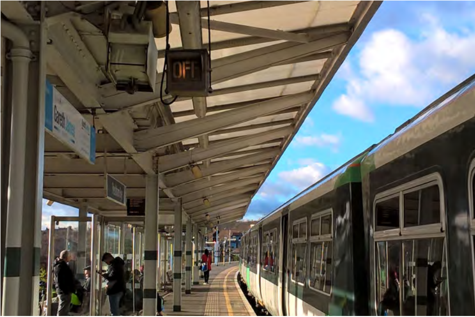
A former BR Southern Region style Off indicator at Peckham Rye, South London. Lit by a filament lamp behind etched glass, the Off aspect was visible when photographed but the station lighting directly above it might make it harder to distinguish.
