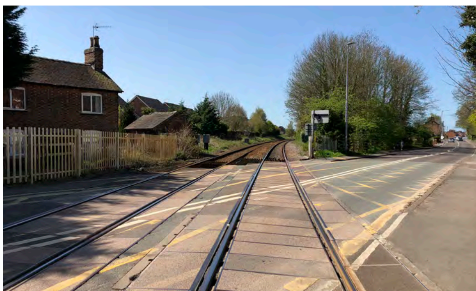
Figure 1 – AHB crossing with a large skew angle making a long walk for crossing pedestrians.
