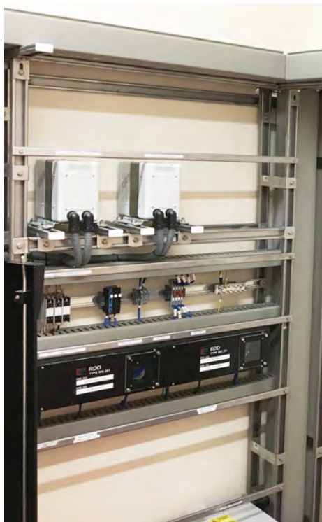
Remote disconnection device trackside (RDD) installation.
