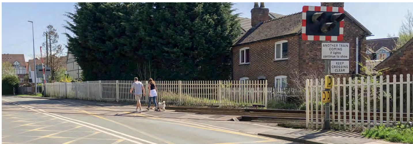
Another view of Newcastle Road, Nantwich. Pedestrians with a dog walk across the AHB crossing with no barrier on the right hand side to prevent access when a train approaches.
