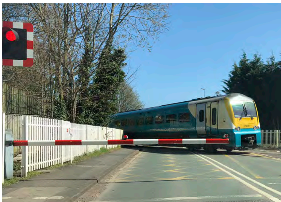
Newcastle Road automatic half barrier crossing, Nantwich. Only a single barrier to stop road traffic and pedestrians.
