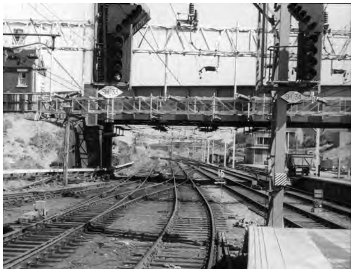
The Crewe-Manchester trial 25 kV electrification was under way in 1958. This picture of the two platform end signals at Sandbach nicely shows the new world of main line signalling; instead of just a 'light on a stick' you had protective screens, guards and all manner of overhead 'knitting'. Photo Westinghouse archive.
