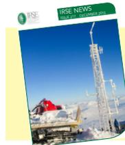
Front Cover: Keeping the trains running over Rannoch Moor on the West Highland line at the White Corries radio site. A team renews the radio antennas and radios used by the Next Generation Radio Electronic Token Block signalling system in the mountains of the highlands of Scotland. *Photo: Lee Clinton, Telnet.*
